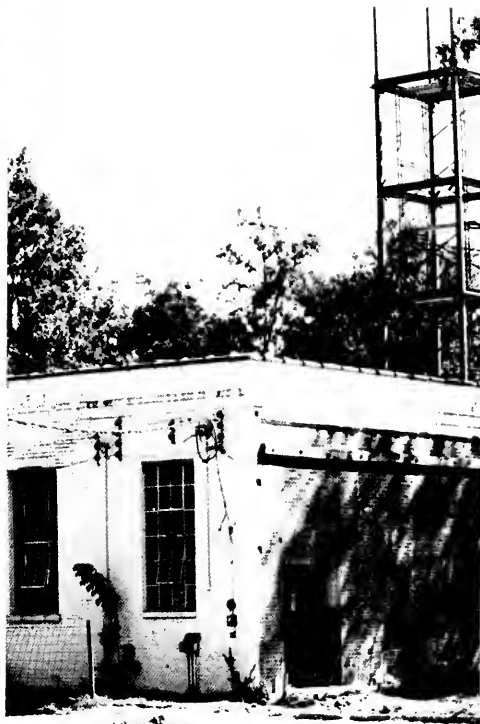
Currently under construction is a new chapel and a campanili.
